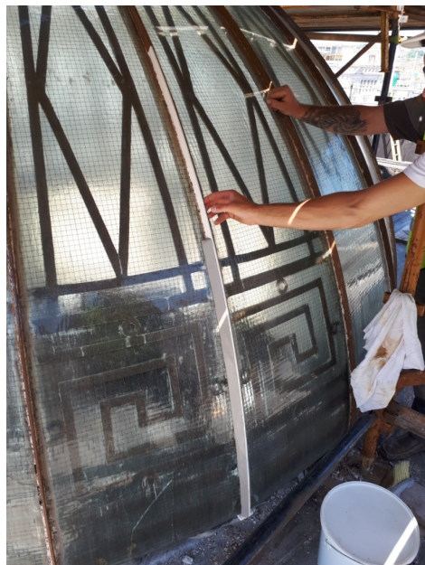
Picture: Works being carried out on dome above Council Chamber
