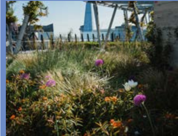
Intensive green roof
