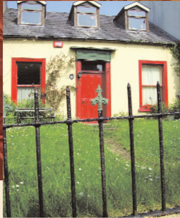
Left: Simple wrought iron railings, Gardiner's Hill
