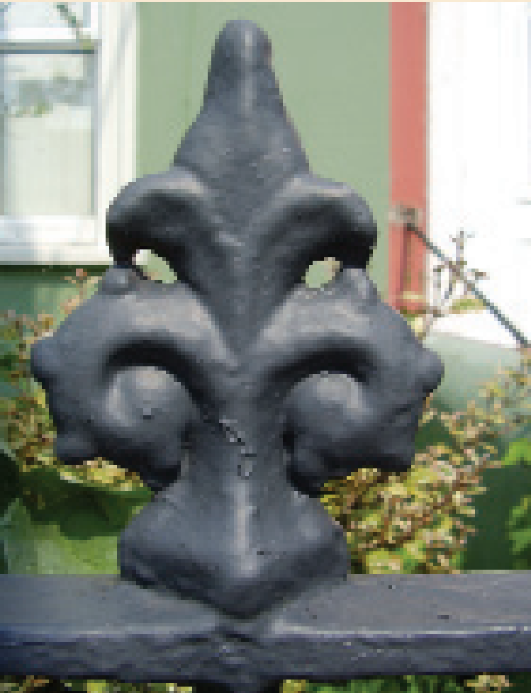
Above: Applying paint too thickly will obscure detail and will reduce the effectiveness of the paint. When paint is applied over corrosion material (rust), corrosion is likely to continue to develop beneath the paint surface
