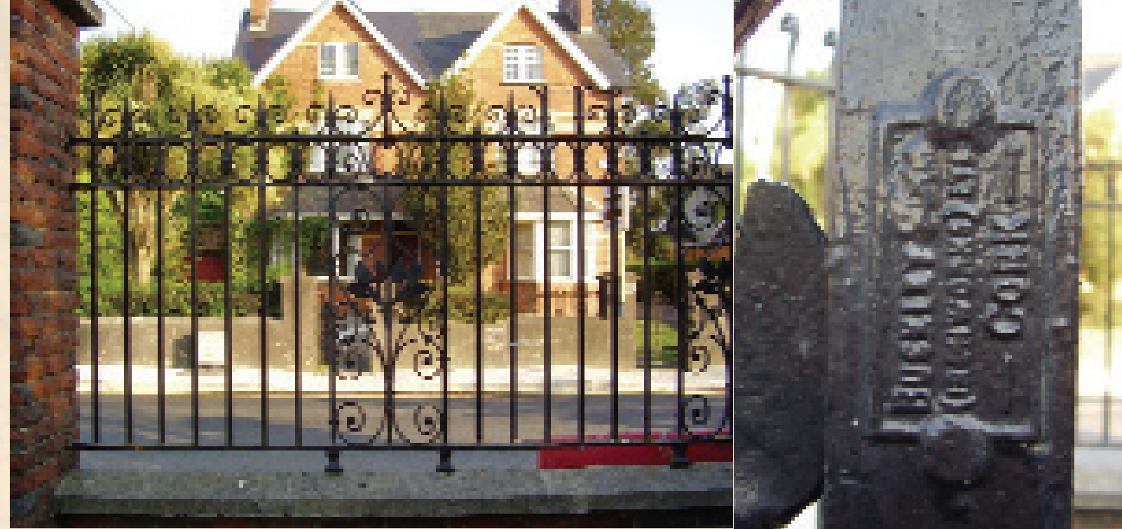
Above: This elegant late 19th Century wrought iron railing, enclosing Bon Secours Hospital on College Road, was made by Buckley & Co (Ironworks) Ltd. of Cork
