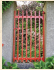
Right: A simple wrought iron gate held together by means of pins and mortise and tenon joints. Military Hill area
