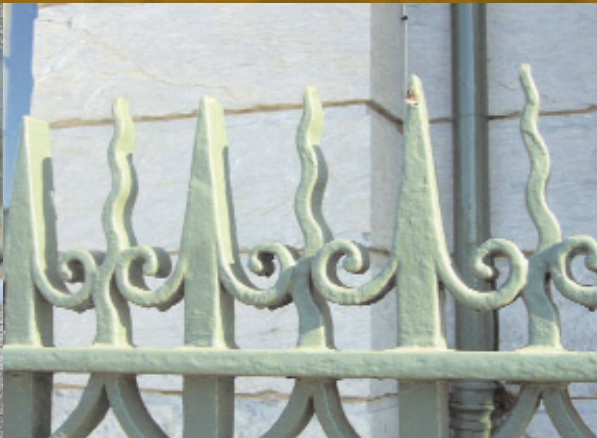
Above: The Georgian style endured with this example on the Old Custom House featuring wavy finials as well as the more ordinary scrolled ones.
