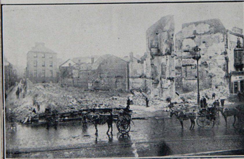
VIEW OF THE RUINS OF MESSRS. CASH & Co.'s PREMISES.
