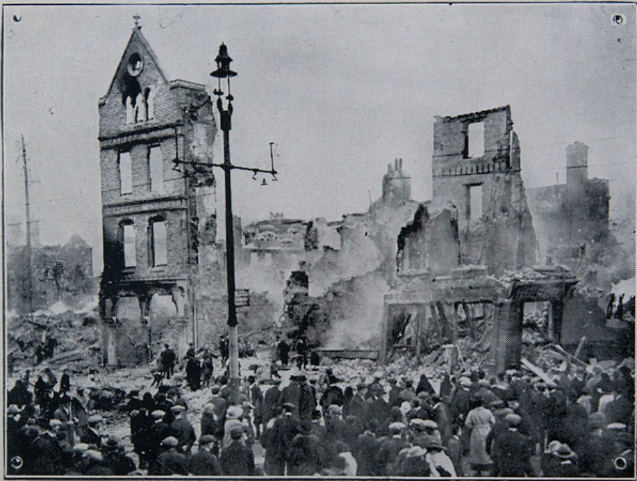
THIS PICTURE SHOWS THE RUINS OF FOUR PREMISES ON THE WESTERN END OF AREA NO. 4
