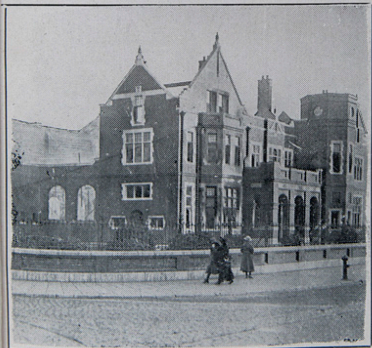
VIEW OF THE CARNEGIE LIBRARY AFTER THE FIRE.
