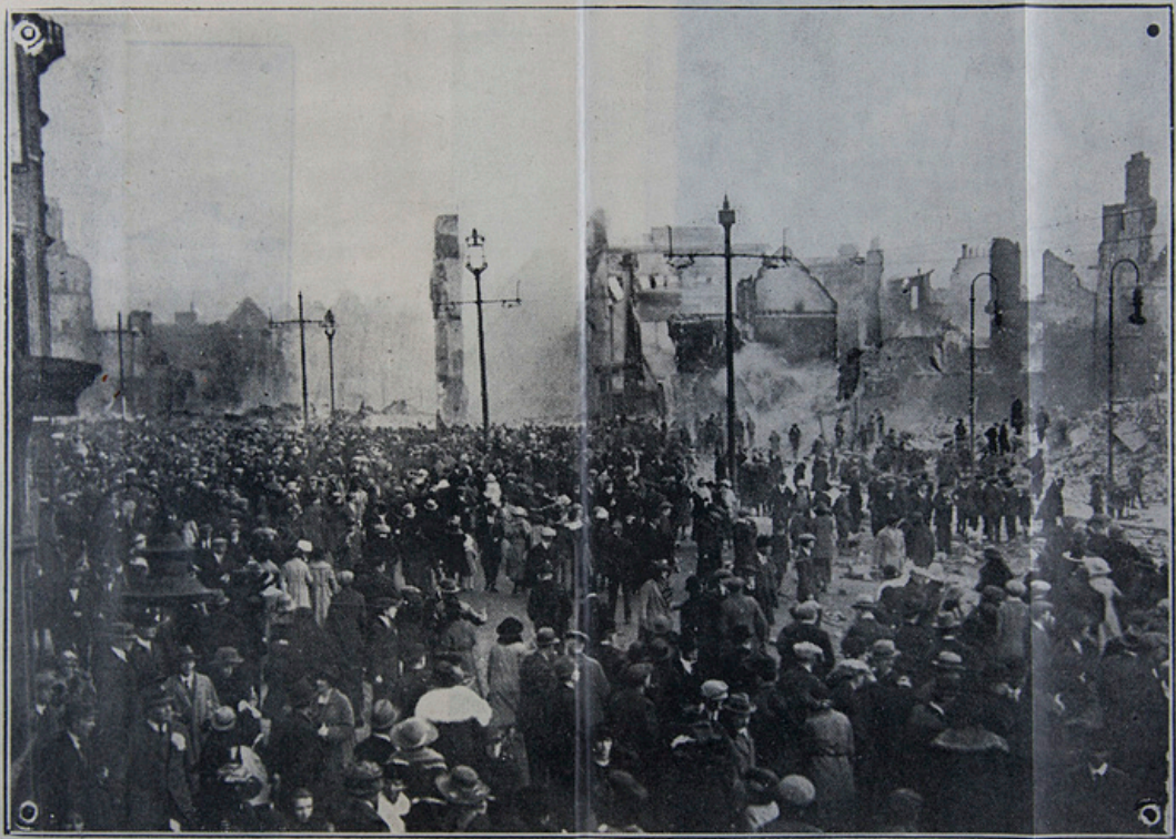
GENERAL VIEW OF THE RUINS OF AREAS 1, 2, 3, AND 4, LOOKING SOUTH.
