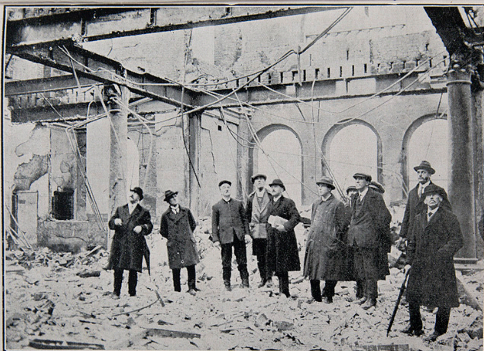
INTERIOR VIEW OF THE RUINS OF THE MUNICIPAL BUILDINGS.
