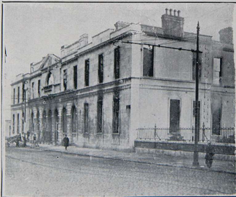
VIEW AFTER THE FIRE.
