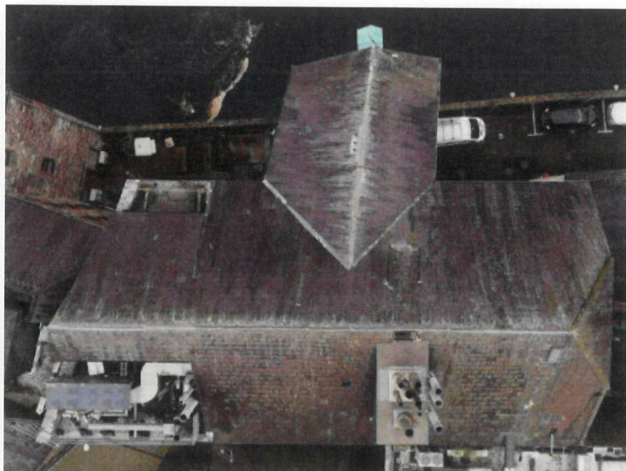
Figure 1: Tyndall Phase 1 Roof. (Image Courtesy of UCC)
