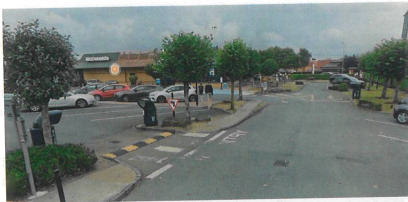
Figure 2: Existing restaurant entrance
