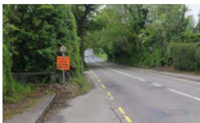
Desire Line 1: Footpath finishes without a safe crossing point to the opposite footpath.
